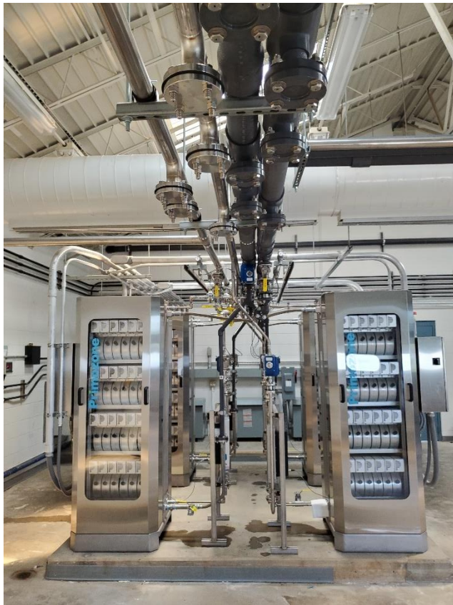
Figure 4. Example of an ozone system (only ozone generators shown).
