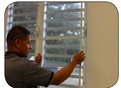
Install or repair window & door screens.
