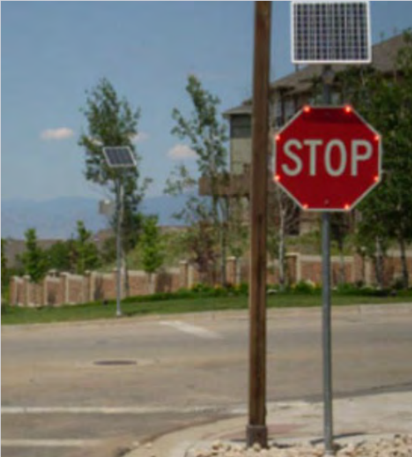
Install Flashing Beacons on Warning Signs
