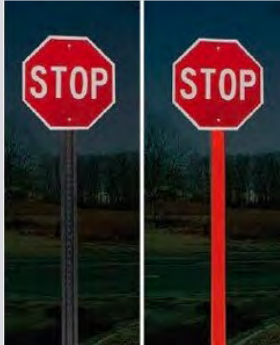
Install Retroreflective Strips on Warning Signs
