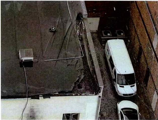
Enlarged View of Building Roof Area 7
