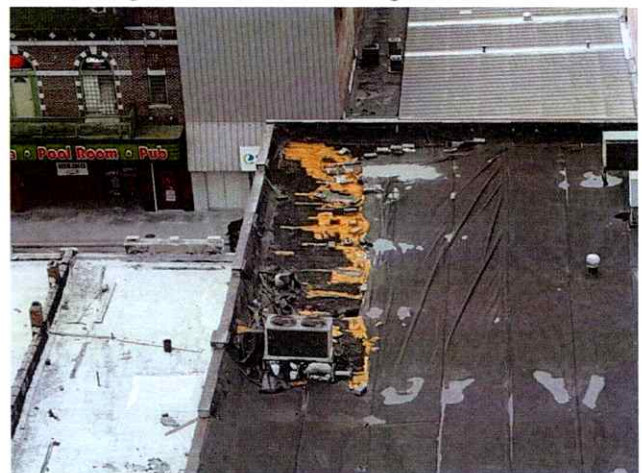
Enlarged View of Building Roof Area 8
