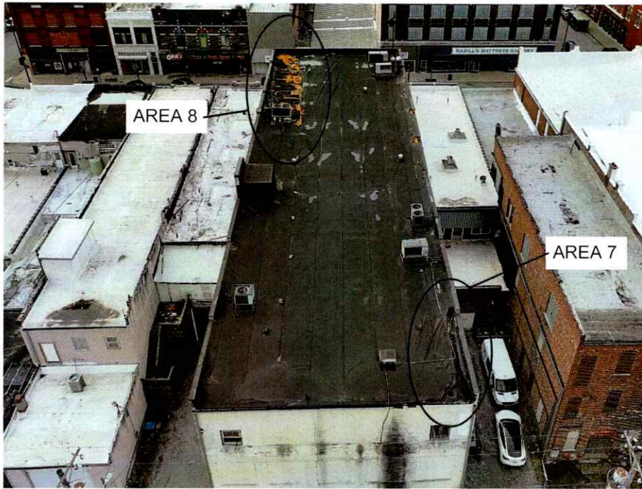
Overall view of building roof.
